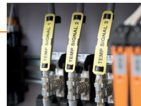
SFX: Highly flexible cable markers – determine the maximum diameter from the length of the cable tie
